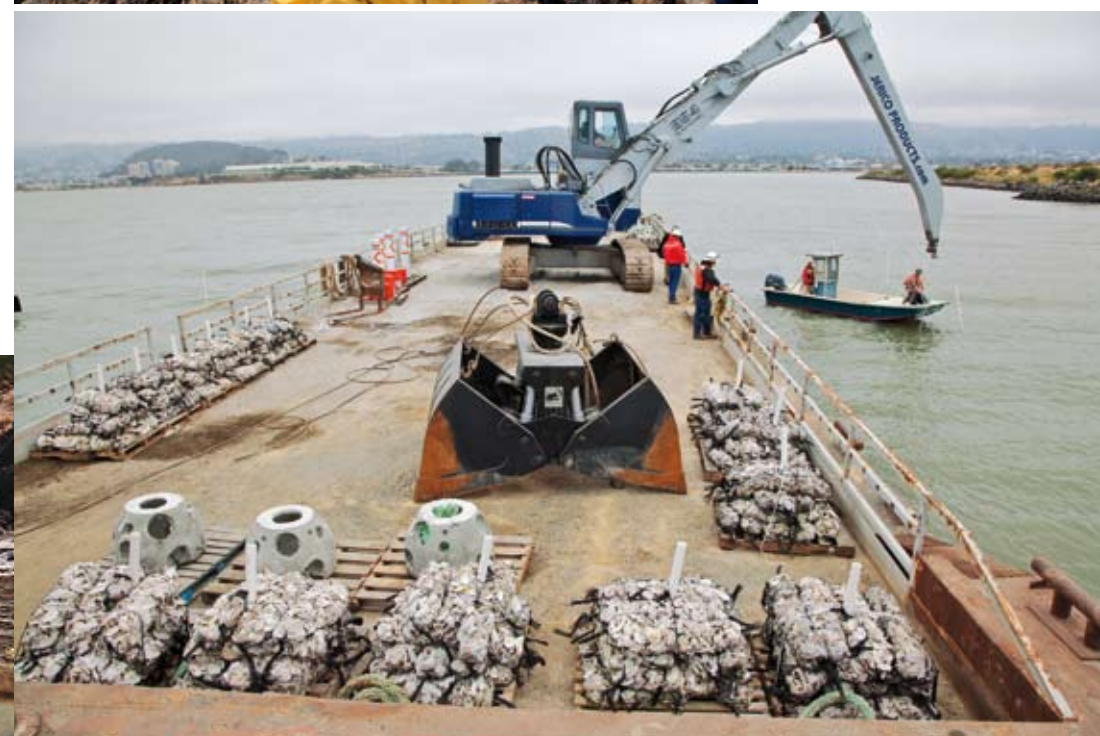
(top right) Bud Abbott has built oyster reefs in Marin and Berkeley. (bottom right) Just off the Berkeley Marina, a crane installs pallets of empty oyster shells where native oysters can settle and create new reefs. (left center and below) Rocky areas are critical anchoring spots for oysters, seaweeds, and other species.
